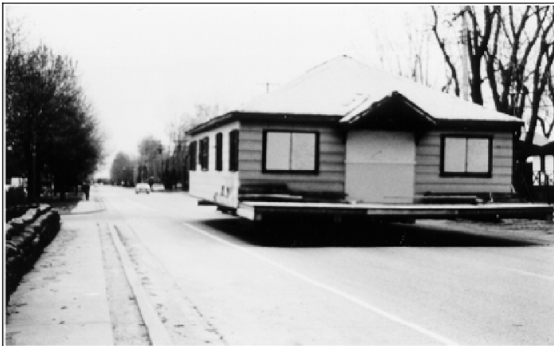
Figure 8.8 Relocation of Residence from Hazardous Lands
