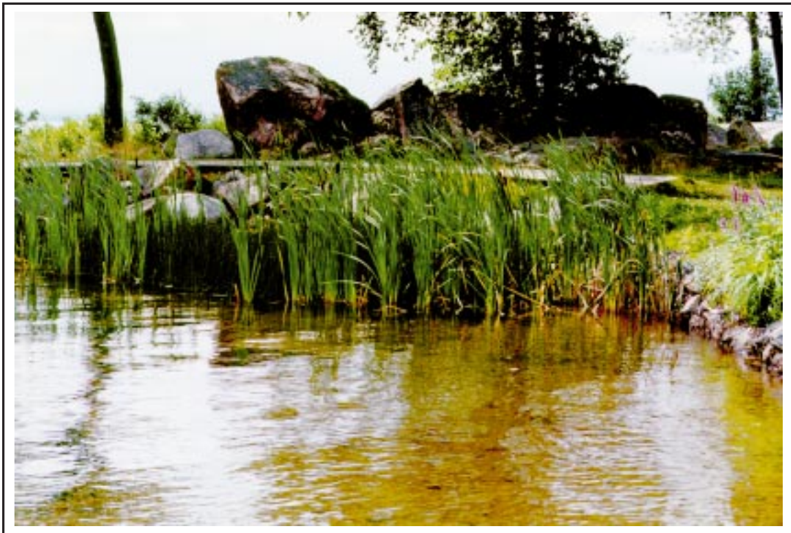
Figure 8.14: Vegetation and Boulders (Biotechnical Approach)
