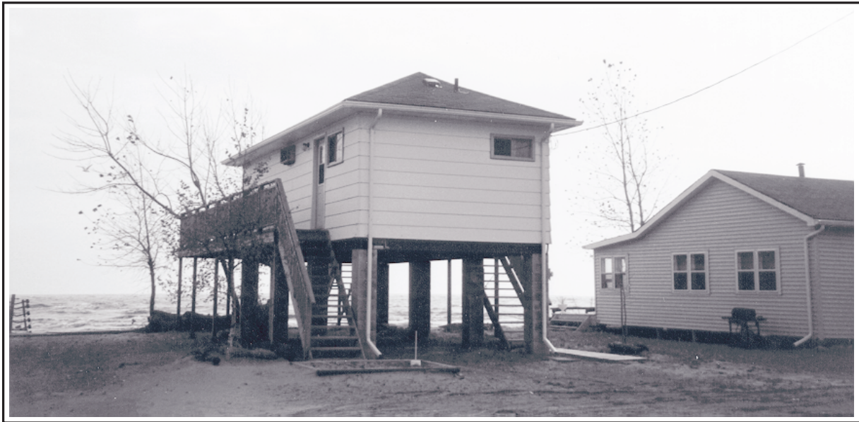
Figure 8.10: Structure Elevated as Floodproofing Measure
