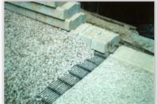
Figure 86 - Drainage Designed by Geotechnical Engineer
