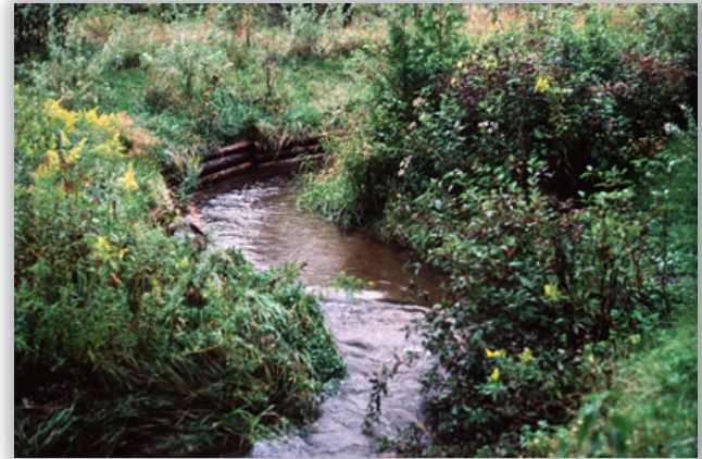
Figure 134 - Log Crib Works
