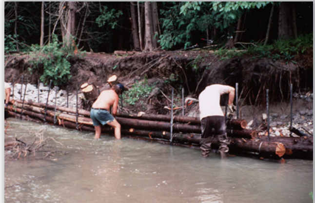
Figure 133 -Installation of Log Crib
