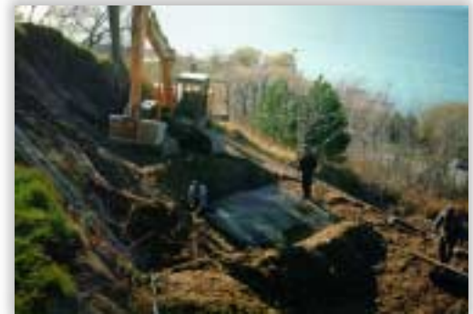
Figure 85 - Installation of Geomattting
