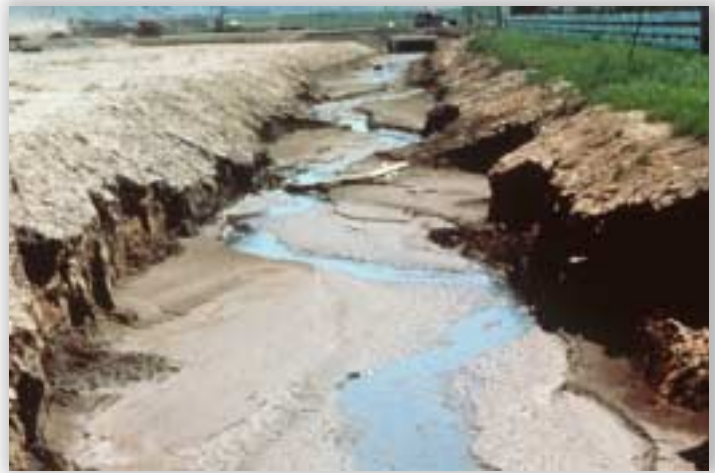
Figure 99 - Example of 'Active' Bank Erosion
